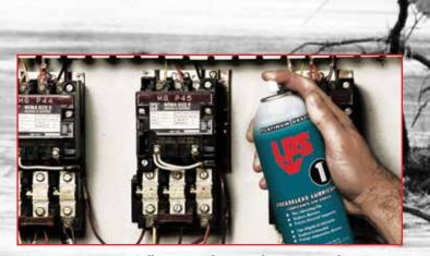
LPS 1® saves potentially water-damaged equipment by penetrating and displacing water allowing a faster start-up. Plus, it cleans, lubricates, and continues to provide greaseless protection that resists dust or dirt.
