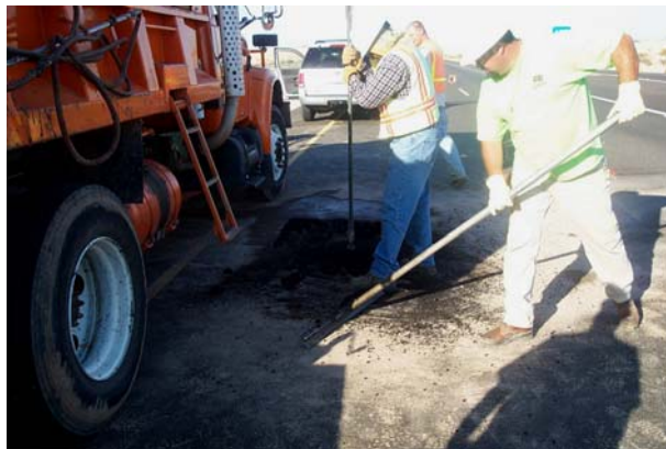
Figure 5-6 Throw and Roll Patching
