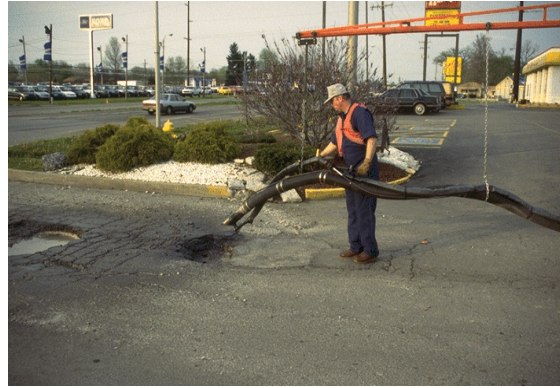
Figure 5-13 Application of Tack Coat
