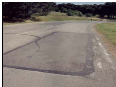
Figure 5-16 Edge Seal Application
