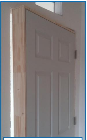
Set the door *roughly* in place: **tuck the hinge- side** of the jamb tight into the frame.
