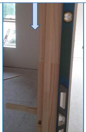
Use a *minimum* of four sets of shims: top and bottom, then two on either side of the *handle*.
