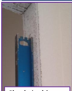
**Check** the hinge**side** of the frame for plumb.
