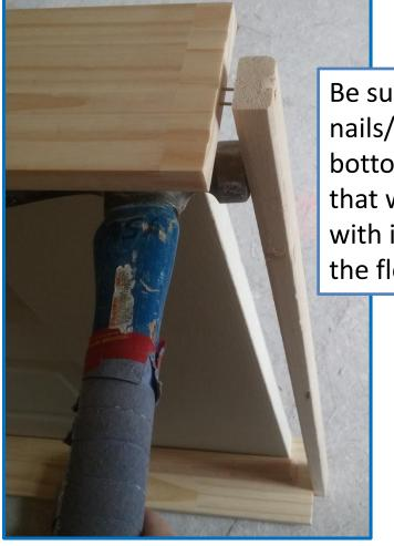
Be sure to remove any nails/staples from the bottom of the jamb that would interfere with it sitting flat on the floor.
