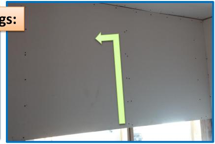
The more screws installed in a sheet, the closer it hugs the framing. Around outlets this can be a problem, but around windows and doors it is a benefit.
