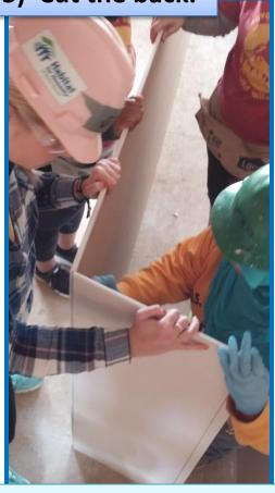
Keeping both pieces of drywall supported, cut the remaining piece of paper along the break line. Make sure all hands are clear of the cut!
