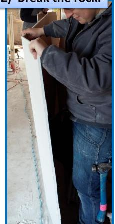
With help, pull the board away from the pile. Push a knee into the back of the cut to break the gypsum along the cut.
