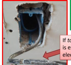
If too much cutting surface is exposed, bit will damage electrical boxes and wires.
