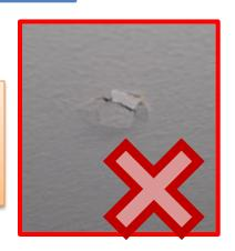
"Nail pops happen because as wood dries, it shrinks. Nails do not shrink. Actually, nails do not pop. The wood shrinks away from the back face of drywall as it dries."
