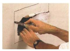
With a drywall saw, cut along the pencil line, then test the patch until it fits.
