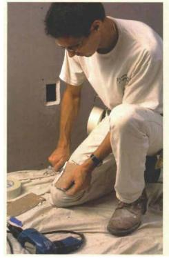
**Bevel edges of the wall opening,** then cut a matching piece and bevel its edges.
