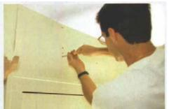
**Refasten drywall** to underlying framing near the popped nail or screw.
