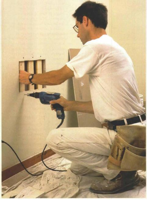
**Furring strips** of 1x2 material will strengthen the repair considerably. Strips should be 6 in. longer than the opening and fastened at both ends with drywall screws.
