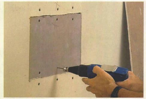
With furring in place, the patch can be attached with drywall screws.
