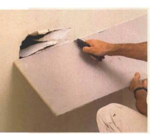
Make a square or rectangular patch slightly larger than the damaged area.
