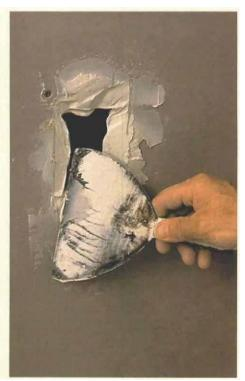
**Add joint compound** to the opening or the patch, then press patch into place.
