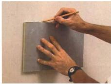
Hold the patch over the damaged area and trace its outline onto the wall.
