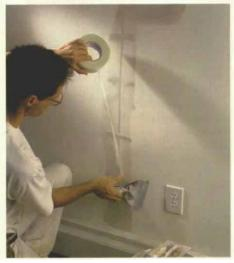
Fill groove with joint compound and apply self-adhering tape over the crack.
